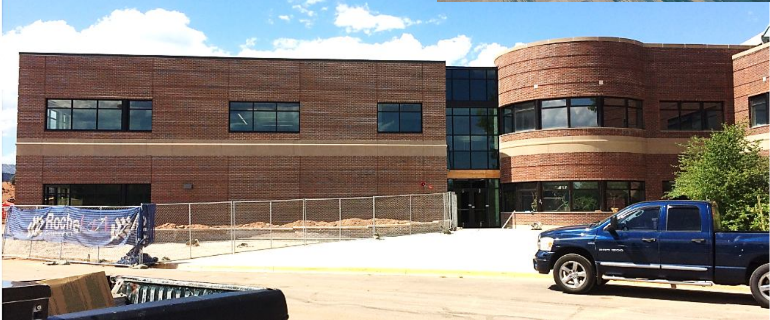
Summit Ridge MS – 8 Classroom Addition
